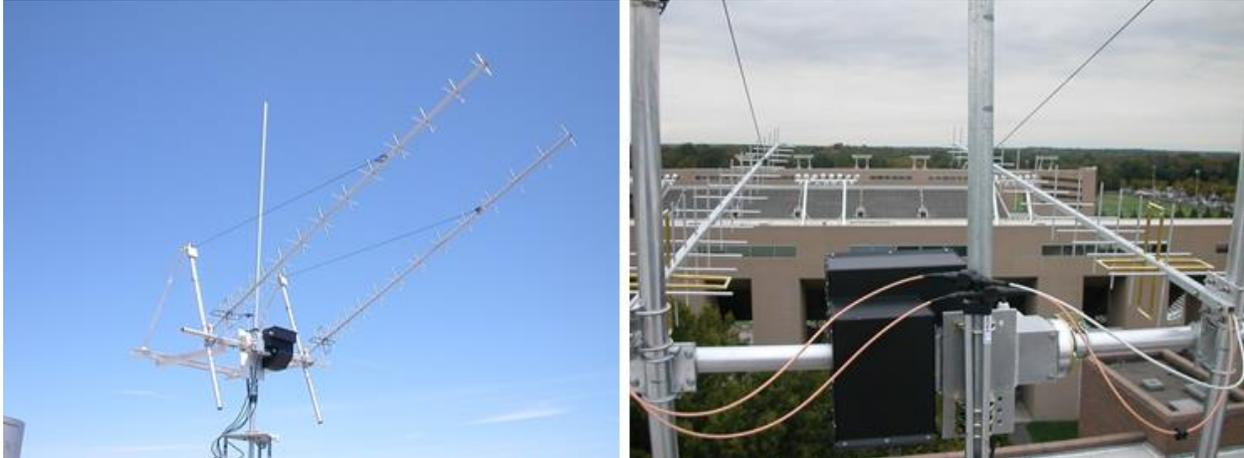
Fig 2. – A pair of 15LFA-JT rear-mounted Yagis on a simple mount with azimuth and elevation control. Separate feedlines carry signals for horizontal and vertical linear polarization from each Yagi to a power splitter. Light-duty dacron ropes serve as forward guys, to prevent boom sag.
